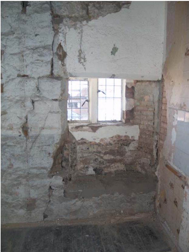
Fig 8: Polesworth Abbey Gatehouse, West range, Tudor fireplace cut by later window
