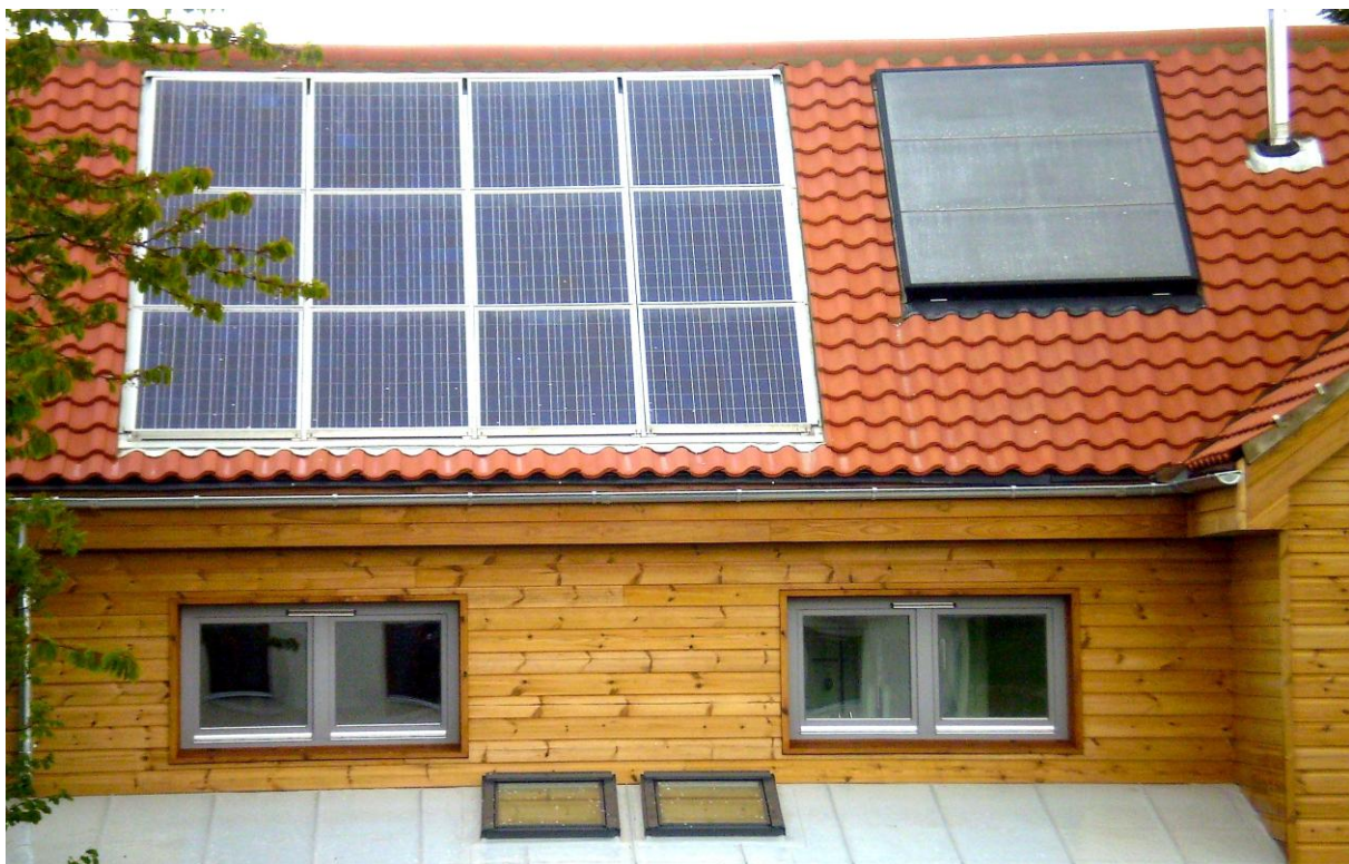
This home at Stawell, built by Ecos Homes using funds raised through Ecos Fund, meets code five of the Code for Sustainable Homes and incorporates PV and solar panels. Image courtesy of Ecos Trust.
