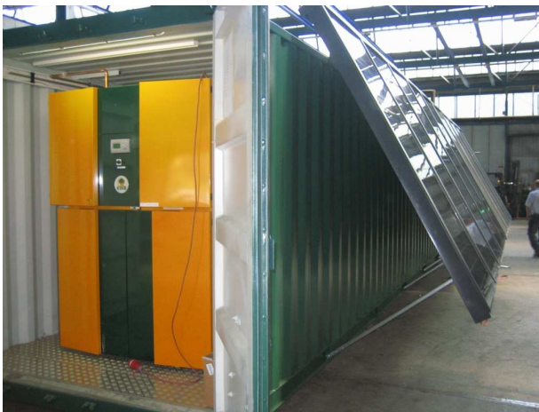
Commercial Energy Cabin with side mounted solar thermal panels Image courtesy of Econergy Ltd/Energy Cabin
