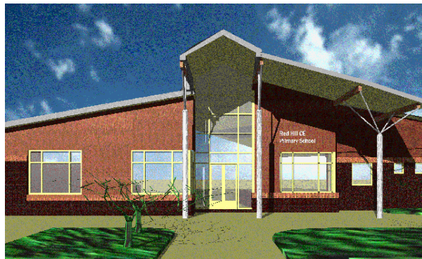
Computer generated image of the main entrance of the new school at design stage
