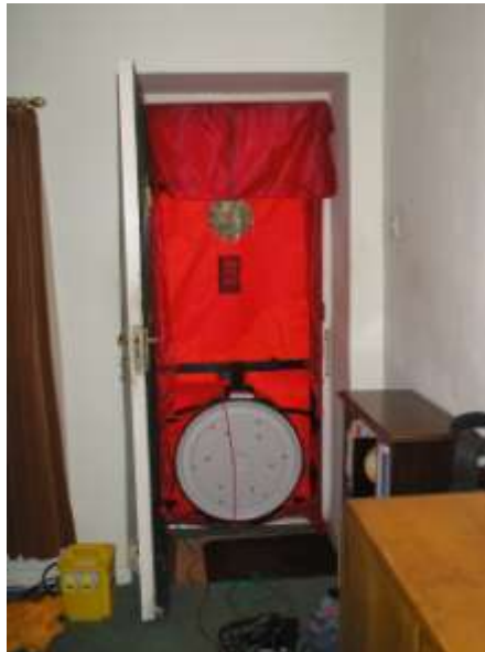
Front door opening with the fan extractor installed
