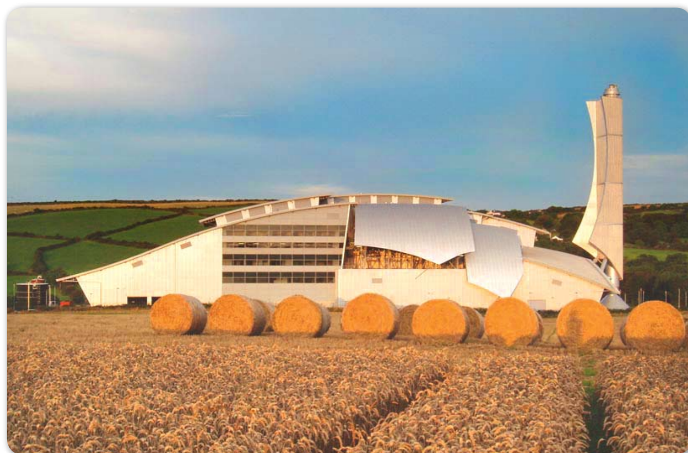
Energy from waste plant – Isle of Man. Photograph courtesy of Sita UK.
